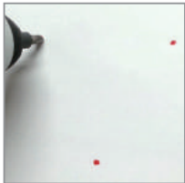
2. Drill 3/16" holes where marked
