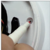
1. Mark screw holes to drill
